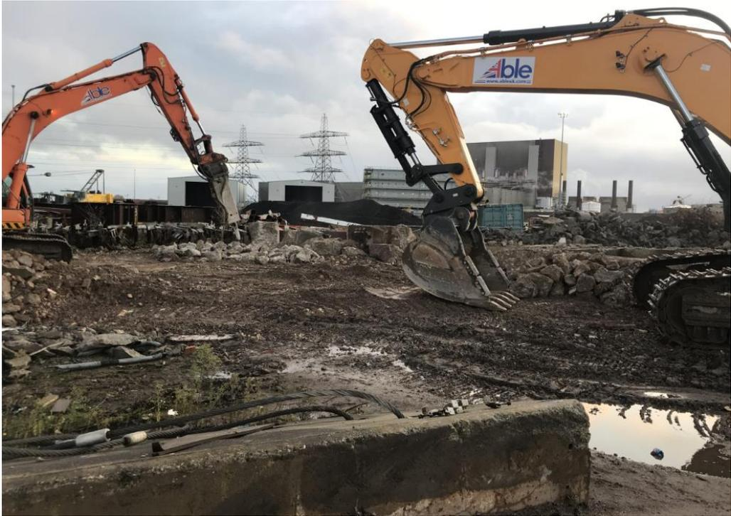
**Plate 3.2 Indicative yellow plant with a bucket (right) and a hydraulic breaker (left) used during construction of Triton Knoll (Source: RWE, 2020)**
