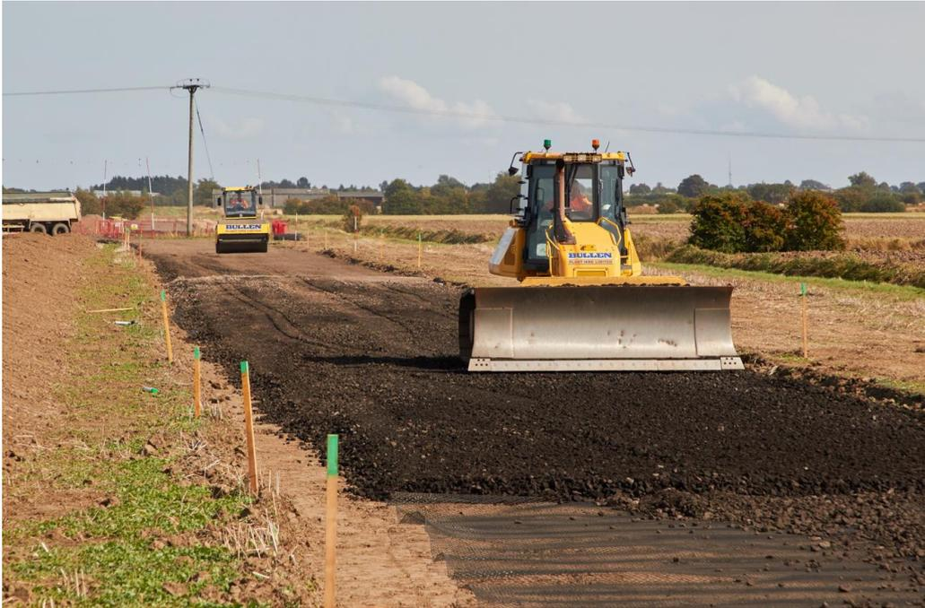
**Plate 3.1 Indicative haul road construction with a bulldozer in the foreground (right) and a roller in the background (left) (Source: Siemens, 2018)**
