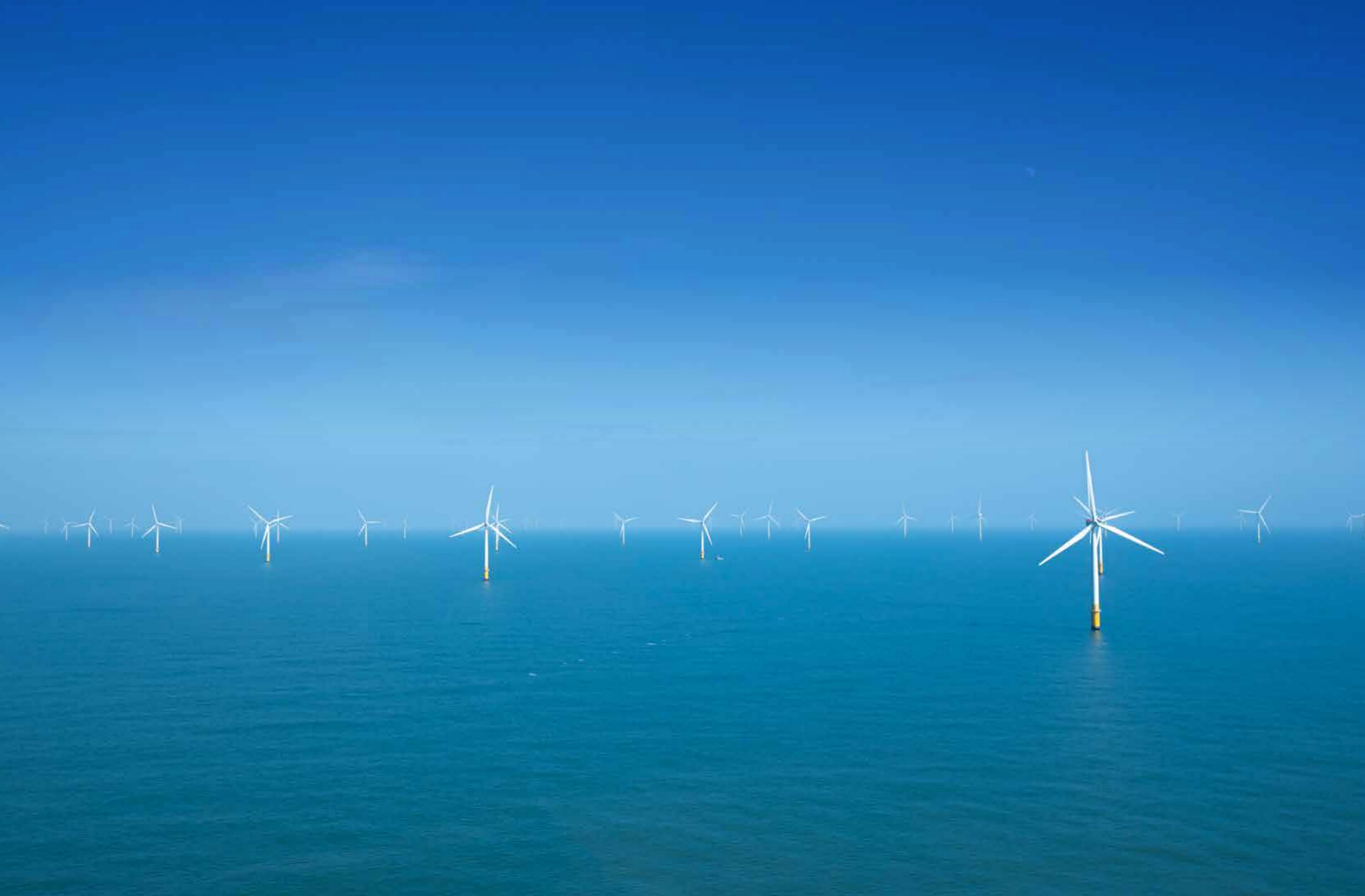
Greater Gabbard Offshore Wind Farm. North Falls' design may differ. Image credit: SSE Renewables.
