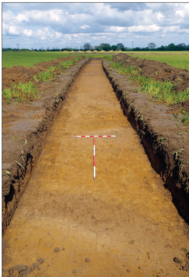
Figure 33: Trench 24, viewed from the north-east
